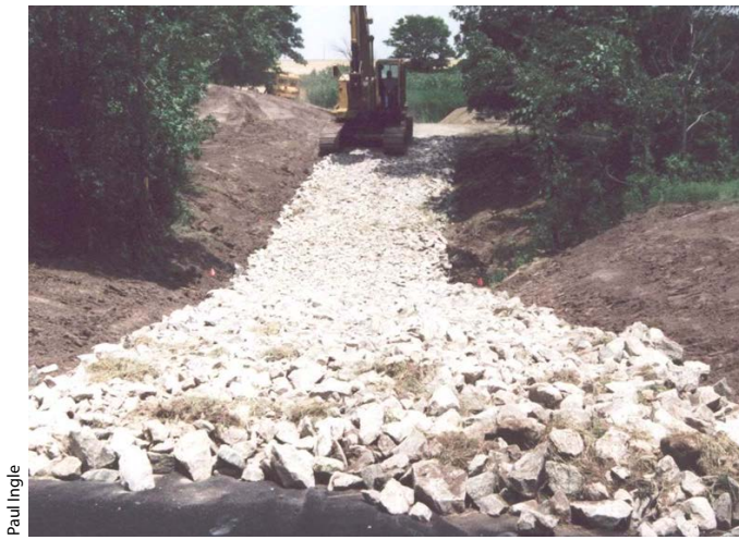
Figure 15. Unvented ford (or hardened stream crossing) under construction. Note the use of geotextile.
