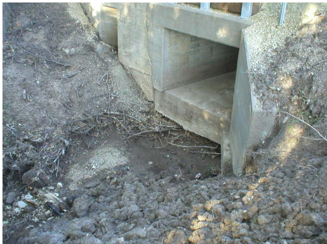
Figure 8. This headcut has reached a box culvert that is now protecting the upstream channel.
