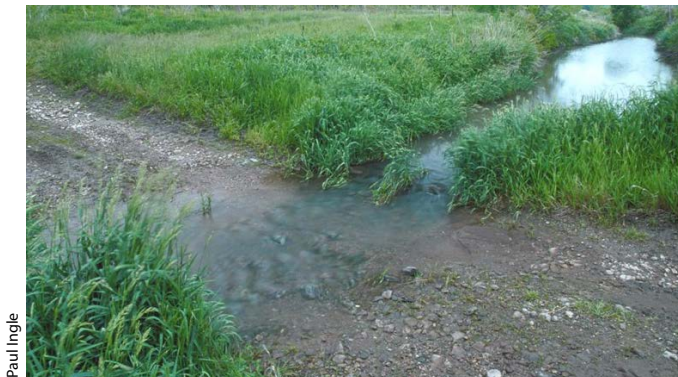
Figure 16. Example of an established hardened stream crossing.
