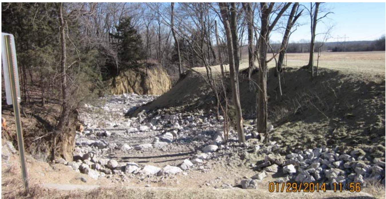
Figure 12. A rock ramp consisting of a series of Newbury Riffles of about 0.5 ft. fall each.
