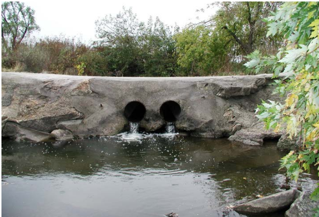
Figure 3. A low water crossing with channel incision or poor design, like this one, creates a barrier to fish and other aquatic organisms.
