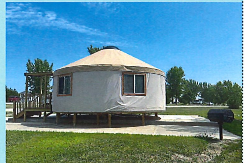
Completed Lookout Yurt Cabin
