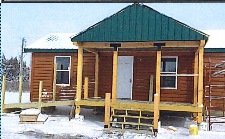
White Rock Cabin, In Progress
